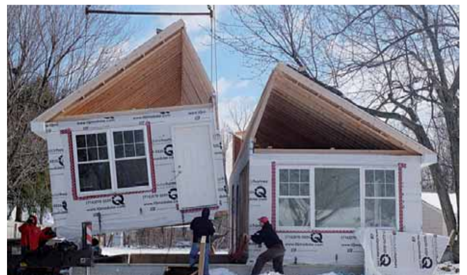
DEPEW, New York: Workers prepare to put together a single-family modular home in Feb 2017. Acquired at tax foreclosure auction, the original home was demolished to make way for new construction by the county land bank. —Reuters
