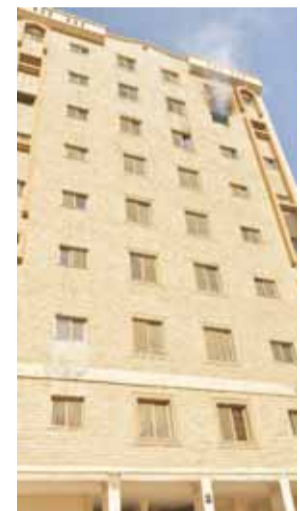
Smoke coming out from a seventh floor apartment in Salmiya.
