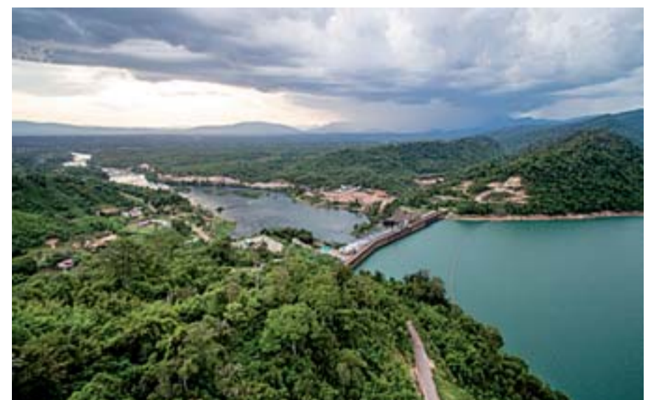
An aerial view of the Nam Ngum hydropower dam, the first built in the nation
