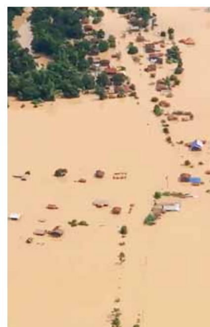
ATTAPU, Laos: This screen grab shows an aerial view of flooded plains yesterday after a dam collapsed the day before. — AFP
