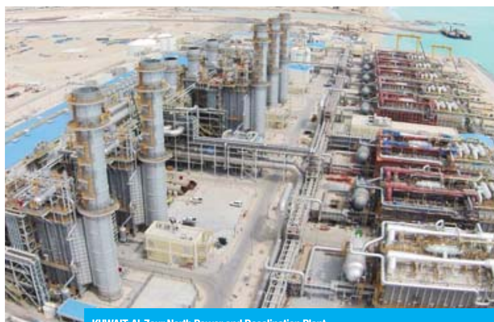
KUWAIT: Al-Zour North Power and Desalination Plant.
