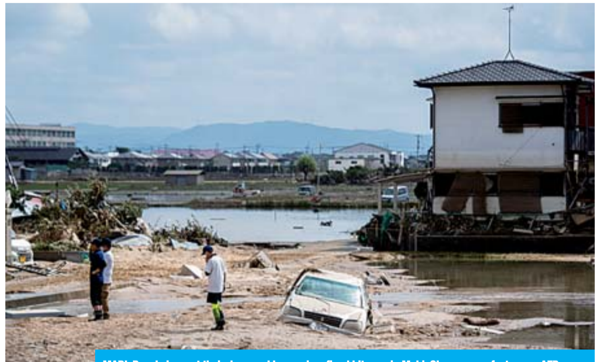
MABI: People inspect their damaged homes in a flood hit area in Mabi, Okayama prefecture. —AFP
