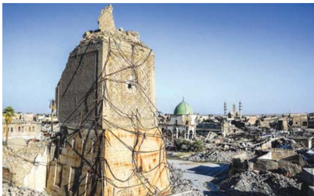
MOSUL: Photo shows a view of the base of the destroyed 'Al-Hadba' leaning minaret, with the dome of the destroyed Al-
