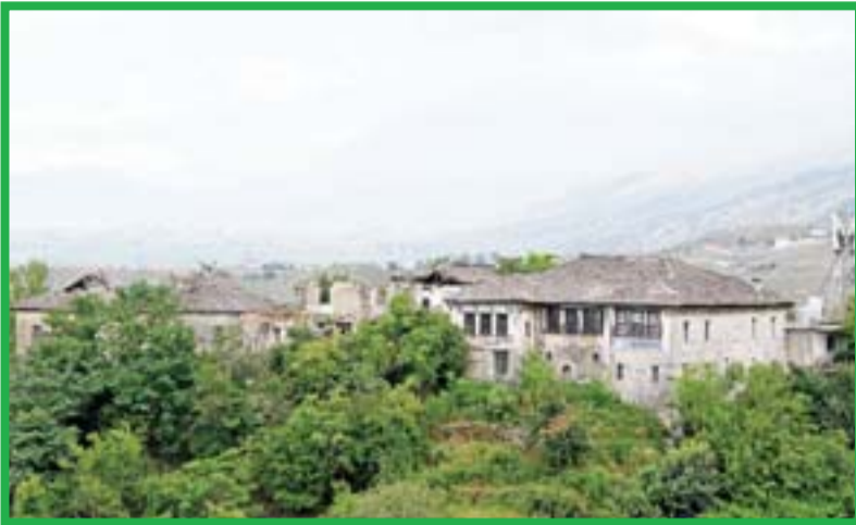
A view of the damaged Karaulli house, in the UNESCO protected city of Gjirokastra.
