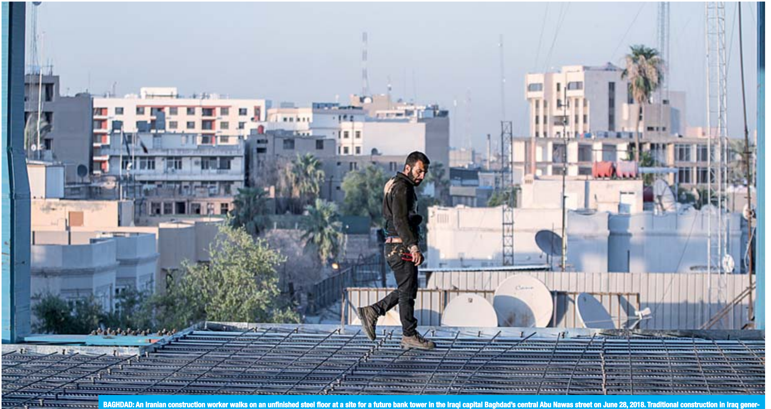
BAGHDAD: An Iranian construction worker walks on an unfinished steel floor at a site for a future bank tower in the Iraqi capital Baghdad's central Abu Nawas street on June 28, 2018. Traditional construction in Iraq generally depends on the use of concrete, as opposed to steel structures which are novel in the country and require Iranian expertise. —AFP
