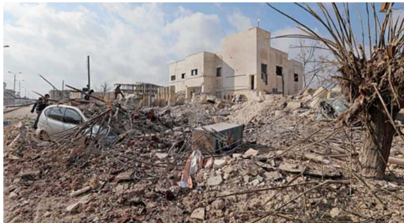
SARAQIB, Syria: Photo shows destruction around the Udai hospital following airstrikes by government forces on the town of Saraqeb in Syria's northwestern province of Idlib. —AFP
