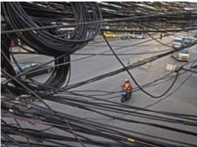
A tangle of cables strung above an intersection in Bangkok.
