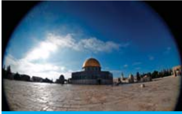
This picture made with a fisheye lens yesterday, shows the Dome of the Rock mosque at the Al-Aqsa mosque compound, in Jerusalem's Old City, following renovation work carried out by the Waqf, a Jordanian-backed body that oversees Muslim religious sites in Jerusalem.
