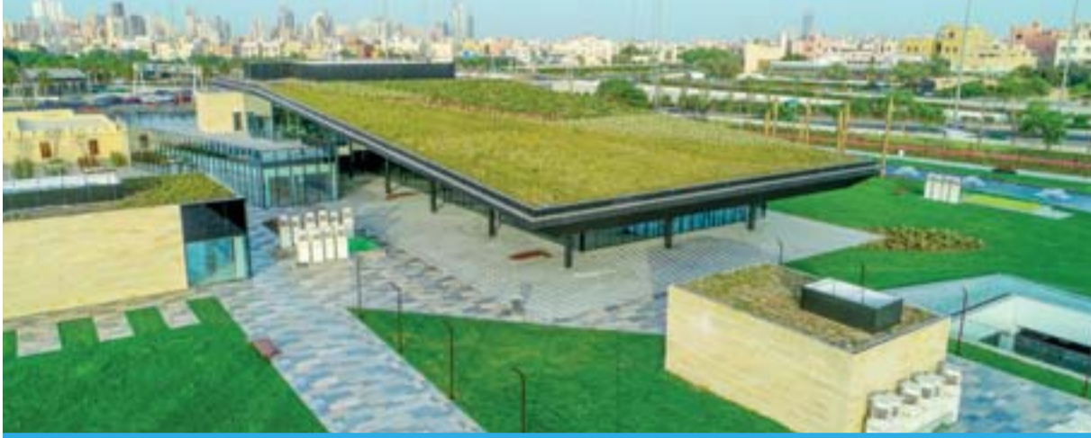
The Green Roofs of the congress center in Al-Shaheed Park (photo courtesy of Al-Hani construction and trading company).
