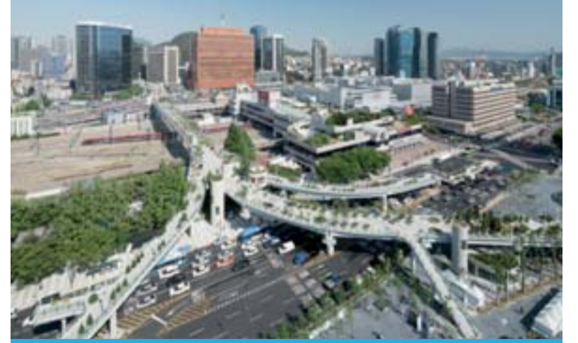
Turning grey into green infrastructures - Seoullo 7017 in South Korea (photo courtesy of Ossip van Duivenbode).
