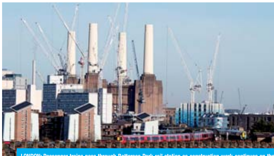
LONDON: Passenger trains pass through Battersea Park rail station as construction work continues on the Battersea Power Station residential and retail development complex in south-west London. —AFP
