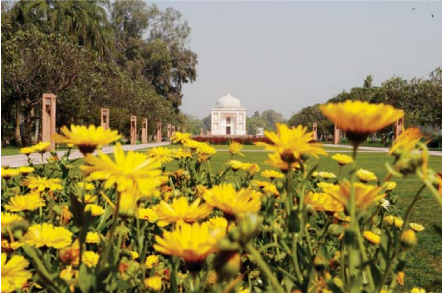
This photo shows the renovated Sunderwala Burj tomb in Sunder Nursery, a 16th-century heritage garden complex adjacent to Indian UNESCO site Humayun's Tomb, in New Delhi. — AFP photos
