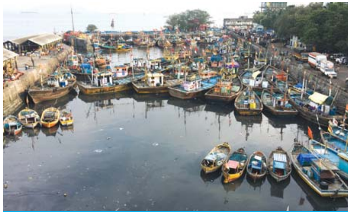
MUMBAI: Sassoon Dock, one of the oldest docks in Mumbai, is set for modernization as part of a planned redevelopment of the city's docklands, the biggest parcel of land to be opened up in the financial hub of India. —Reuters
