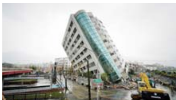
HUALIEN, Taiwan: Rescue workers block off yesterday the area outside a building which tilted to one side after a strong quake rocked eastern Taiwan. — AFP
