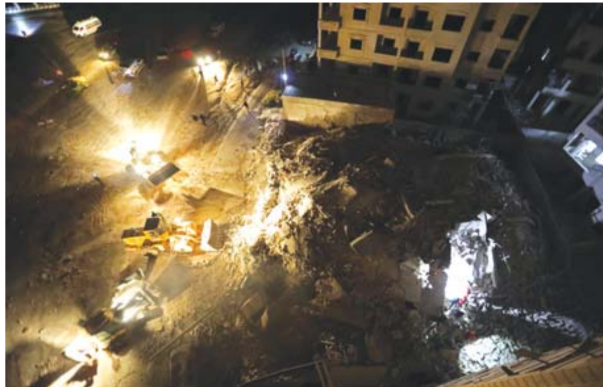
IDLIB, Syria: Syrian emergency services search for members of four families reportedly stuck under the rubble of a six-storey building that collapsed following Syrian government air strikes in Idlib. —AFP
