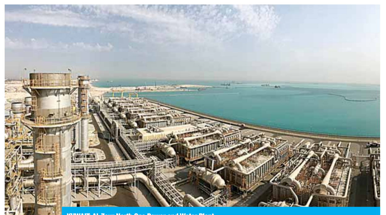
KUWAIT: Al-Zour North One Power and Water Plant.
