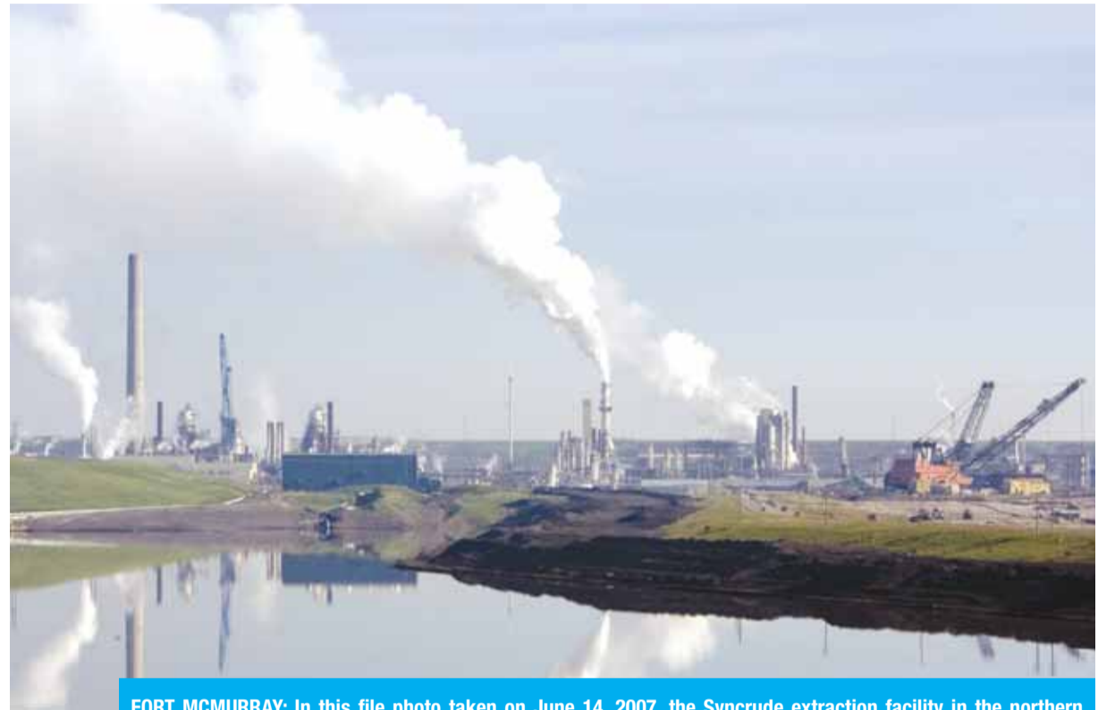
FORT MCMURRAY: In this file photo taken on June 14, 2007, the Syncrude extraction facility in the northern Alberta oil sand fields is reflected in the pool of water being recycled for re-use in the extraction process in Fort McMurray, Alberta, Canada.
