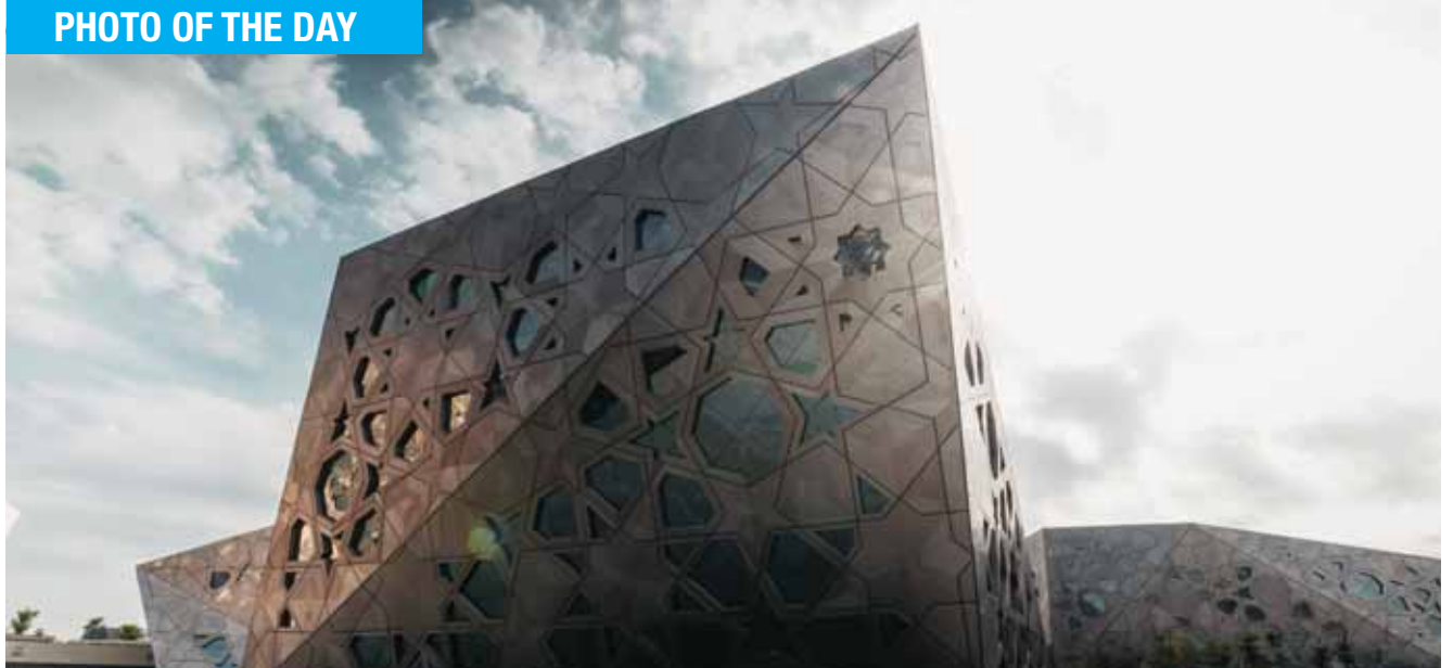
Photo shows the architectural details of the facade of the Sheikh Jaber Al-Ahmed Al-Sabah Cultural Center in Kuwait City. — Photo by Yassine Bensaid/KUNA
