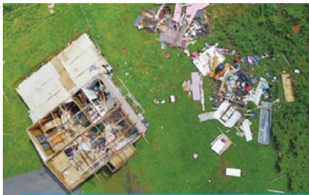
PUERTO RICO: A house destroyed by hurricane winds is seen in Barranquitas, southwest of San Juan, Puerto Rico, following the passage of Hurricane Maria. — AFP
