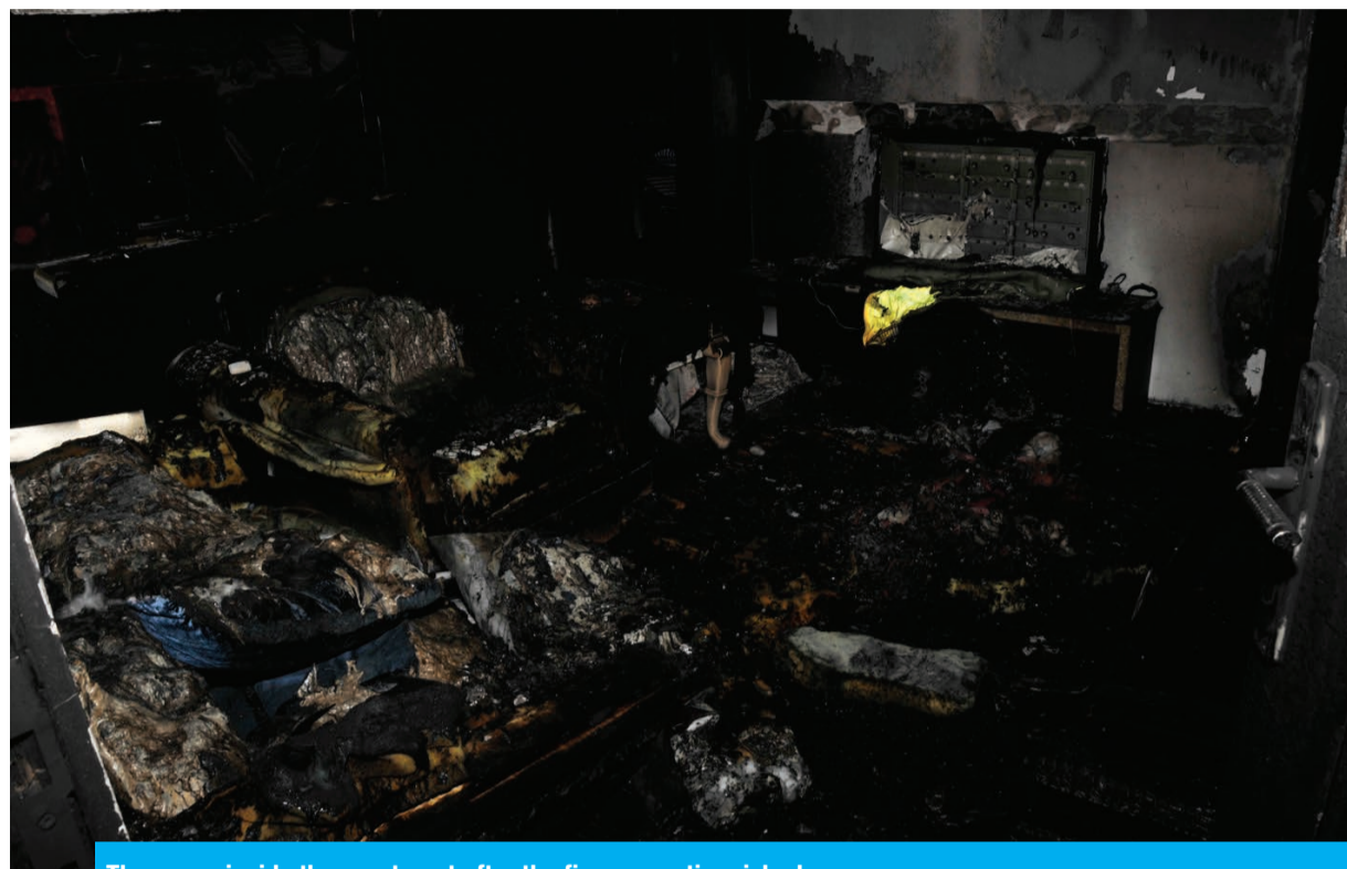
The scene inside the apartment after the fire was extinguished.
