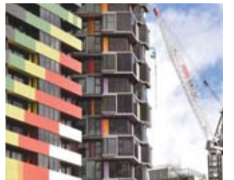
MELBOURNE: A crane works next to an apartment building in Melbourne yesterday. Australia marked two years since it last moved interest rates by keeping them on hold again yesterday with stubborn wage growth and high household debt continuing to weigh on sentiment. — AFP
