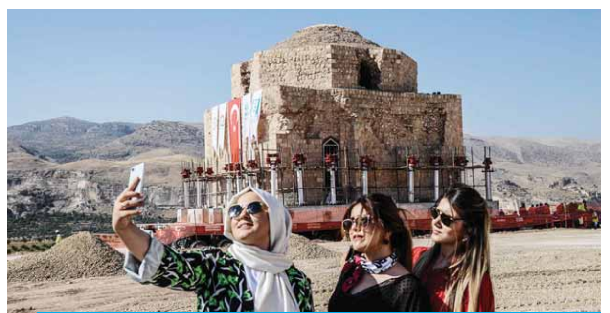
HASANKEYF, Turkey: Women take a selfie as the Artuklu Hamam, a centuries-old bath house weighing 1,600 tons, is loaded onto a wheeled platform and moved down a specially constructed road yesterday. — AFP
