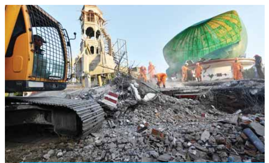
PEMENANG, Indonesia: Indonesian search and rescue personnel work on a collapsed mosque in North Lombok yesterday, a day after a 6.9 magnitude earthquake struck the area. — AFP
