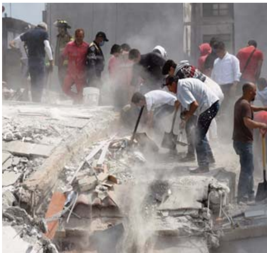
MEXICO CITY: People hurry to free possible victims out of the rubble of a collapsed building after a quake rattled Mexico City yesterday. — AFP
