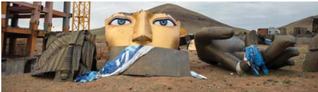
This picture shows the construction site of the Grand Maitreya Spiritual Centre on the outskirts of Ulan Bator. — AFP photos
