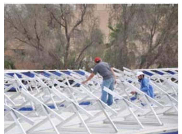
Workers are seen at the project's site.
