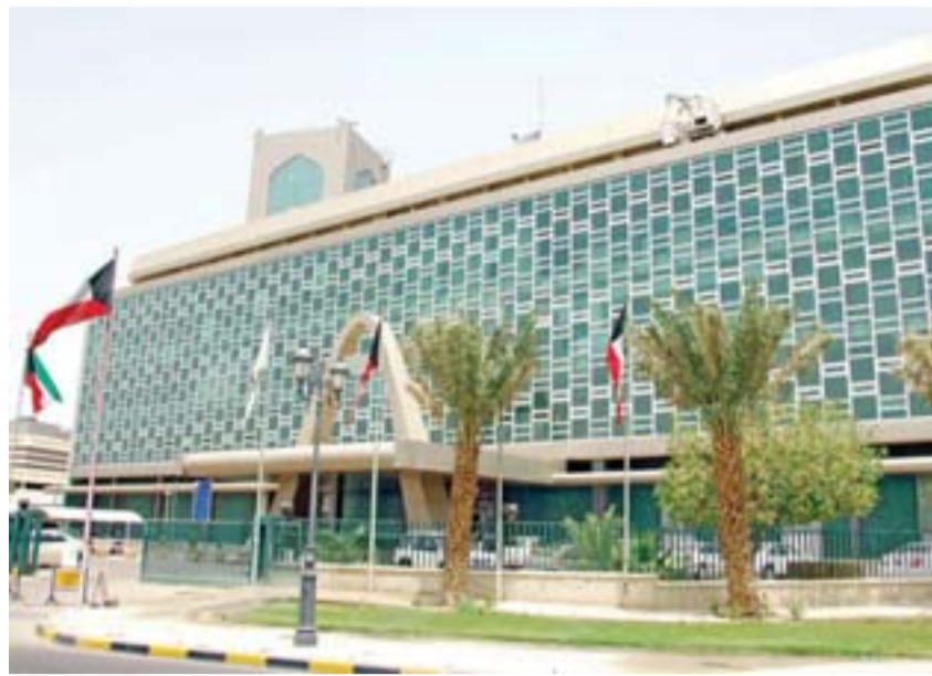
The Municipal Council's building.
