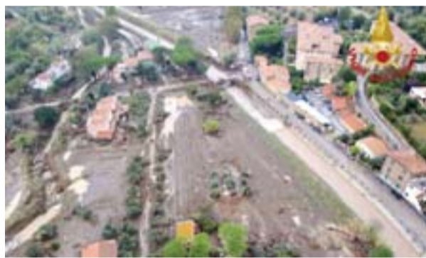
ITALY: An aerial view of the city of Leghorn, Italy, following floods. — AP
