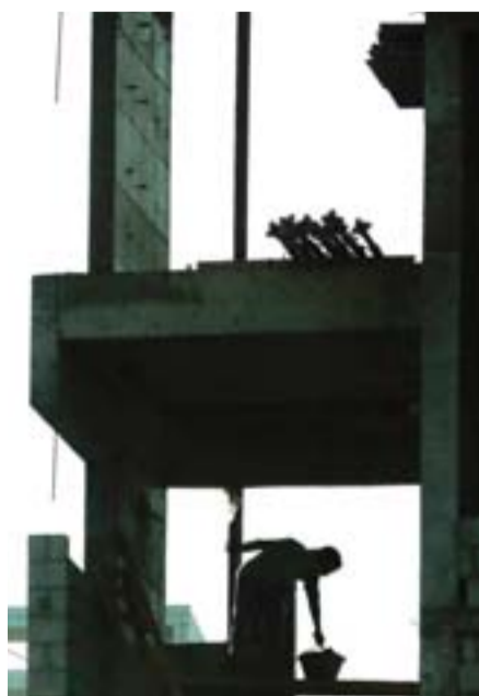
KUWAIT: A worker is seen at a construction site yesterday. — Photo by Yasser Al-Zayyat
