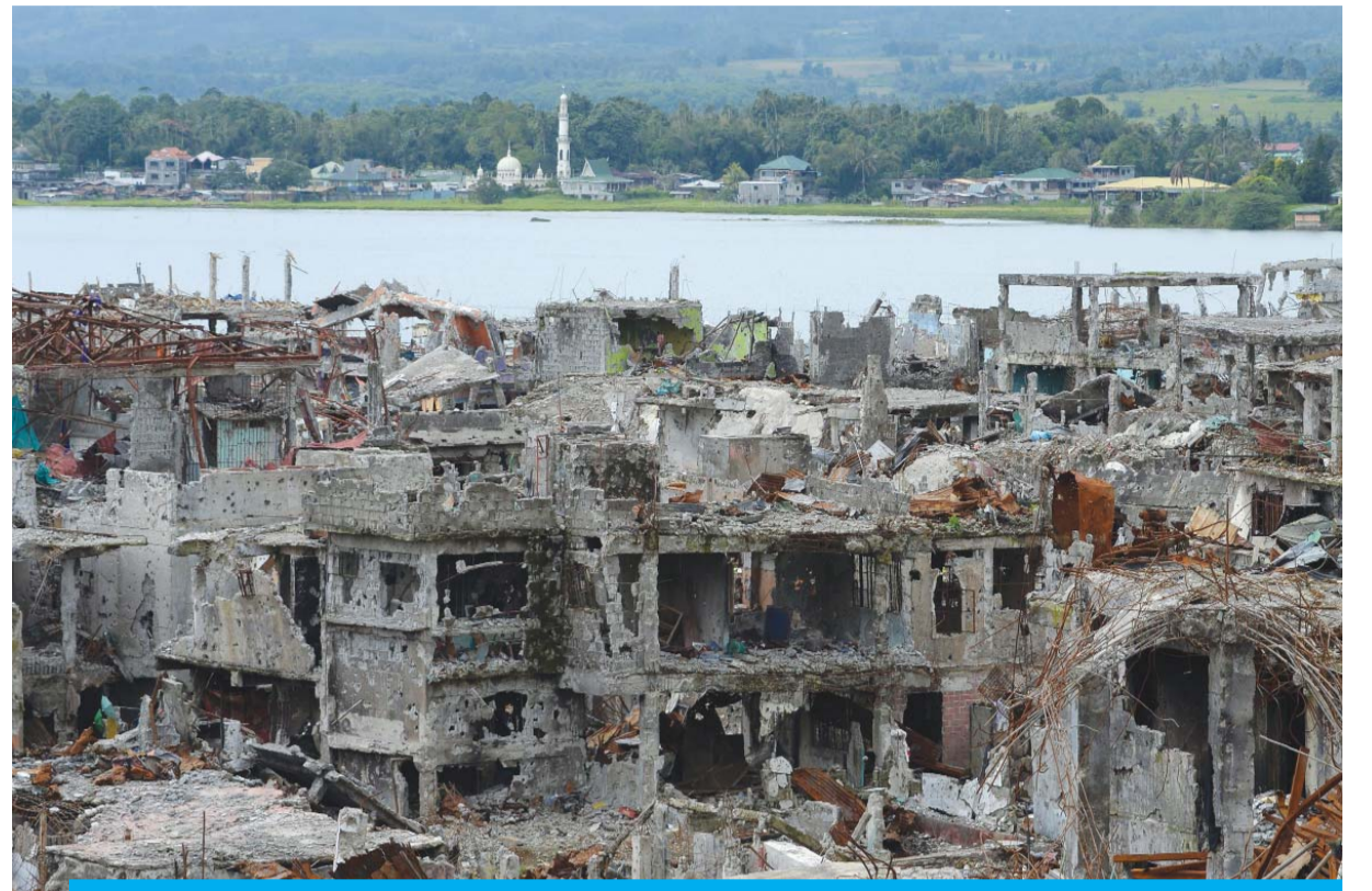
MARAWI: Photo shows bombed-out buildings inside the main battle area between government troops and IS-inspired Muslim militants in Marawi. —AFP
