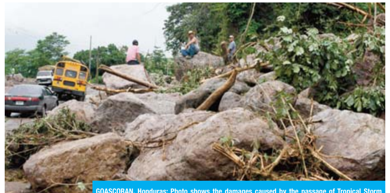
GOASCORAN, Honduras: Photo shows the damages caused by the passage of Tropical Storm Nate, near Goascoran, in Valle department, Honduras. — AFP
