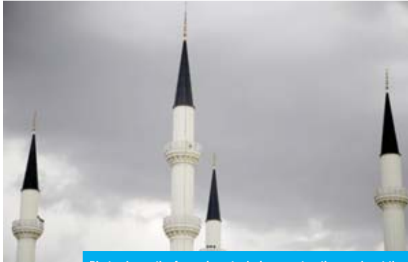
Photo shows the four minarets during construction works at the Hala Sultan mosque outside of the divided capital Nicosia, in the Turkish occupied northern part of the Island of Cyprus. — AP
