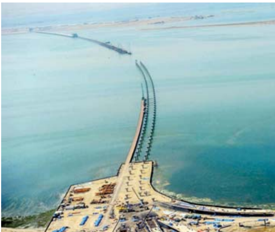
KUWAIT: Aerial view of the Sheikh Jaber Al-Ahmad Causeway Project.
