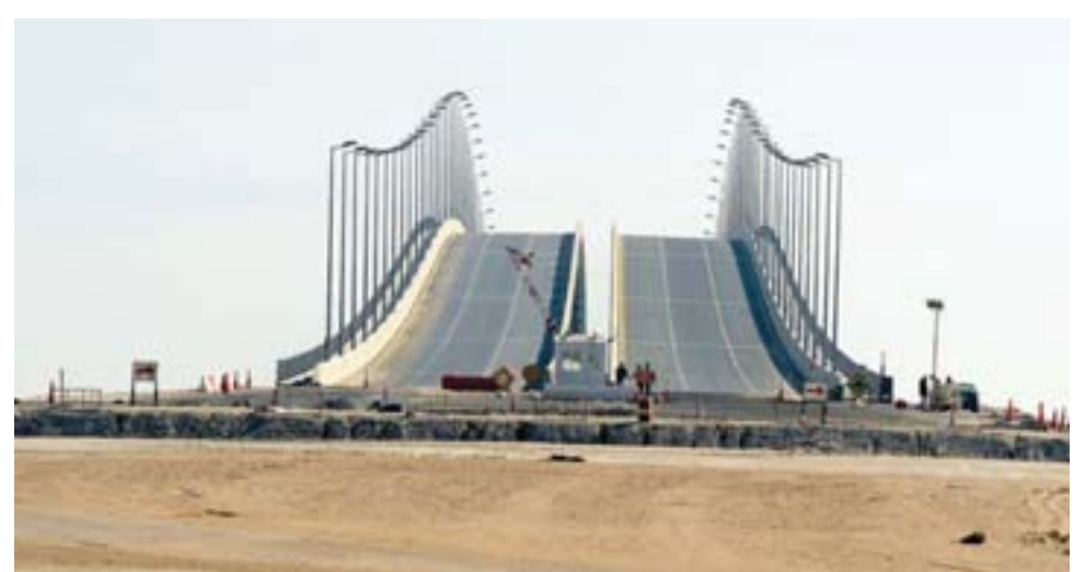
Construction works for a bridge connecting Boubyan Island with the mainland, built as part of the Mubarak Al-Kabeer Port mega project.
