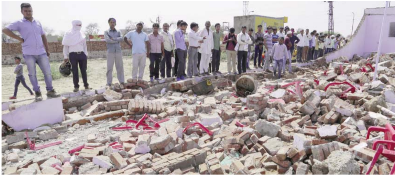
BHARATPUR, India: People look at the debris after a building wall collapsed onto guests at a wedding in this district in Rajasthan state yesterday. — AP
