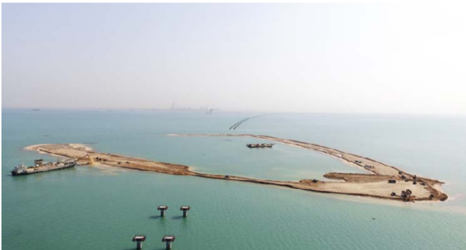
Construction works at the Jaber Causeway project.
