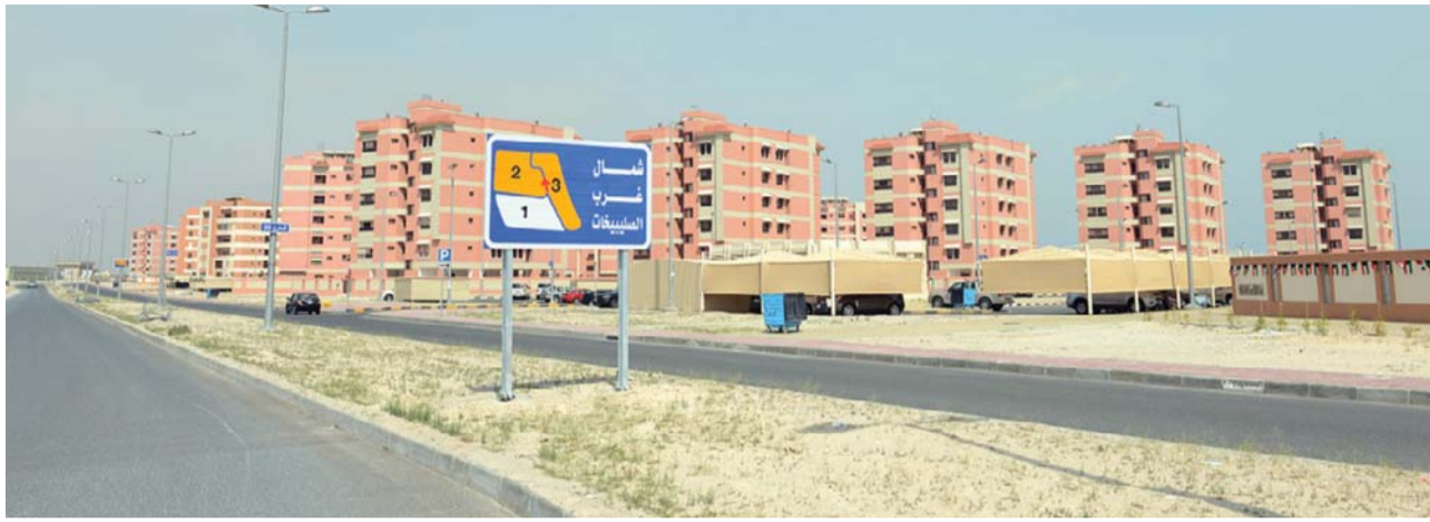
Sabah Al-Ahmad housing project
