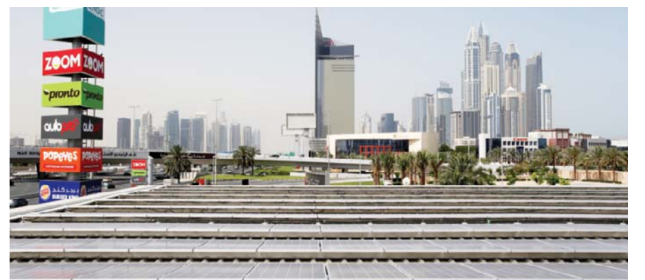
DUBAI: Solar panels power an Emirates National Oil Company gas station, in Dubai, United Arab Emirates. The government-owned oil company said the country's first solar-powered gas station in Dubai, on the city's main Sheikh Zayed Road thoroughfare, is covered with solar panels that can generate up to 120 kilowatt hours. — AP
