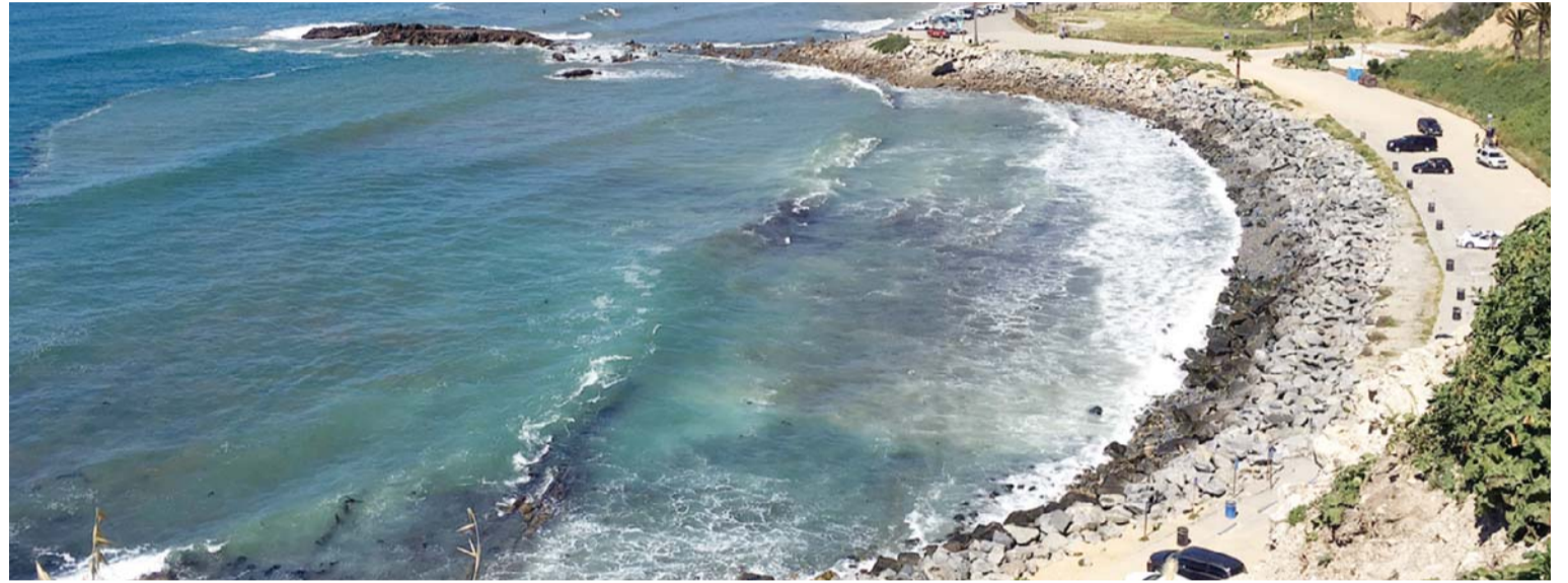
LOS ANGELES: In this photo, Royal Palms Beach in the San Pedro area of Los Angeles is protected by boulders placed there to forestall erosion. — AP
