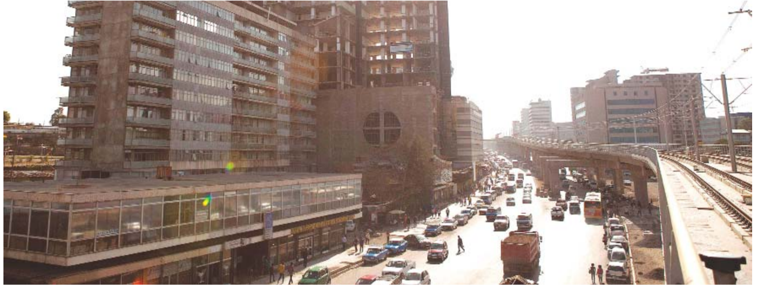
ADDIS ABABA: This file photo taken on April 3, 2015 shows view due west from the Meskel Square station of the Addis Ababa light rail. Electric light railway tracks soar over Ethiopia's capital, a rare example of mass transit infrastructure on a continent ruled by ramshackle, diesel-spewing buses.
