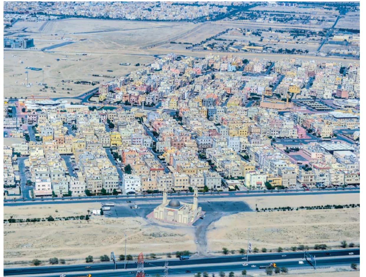
Homes in the Saad Al-Abdullah residential project.
