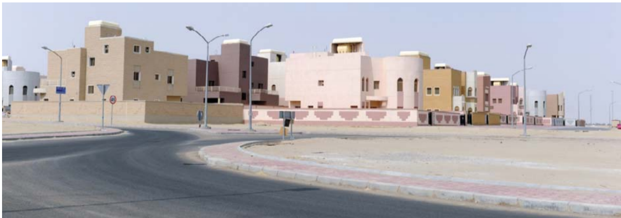
Sabah Al-Ahmad housing project.
