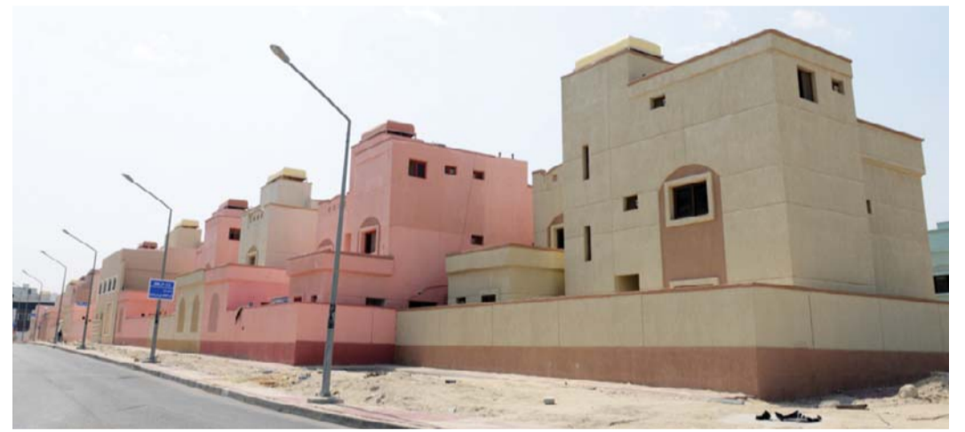
Housing projects northwest of Al-Sulaibkhat.
