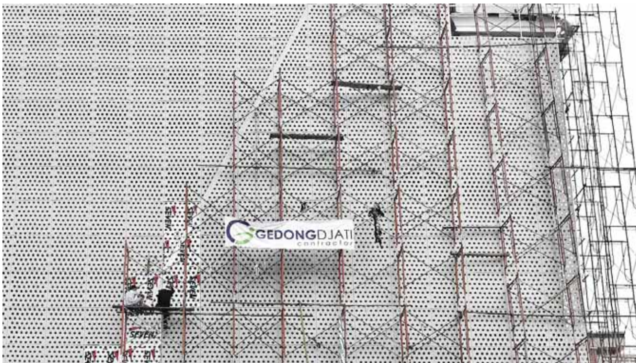
JAKARTA: Workers install building glass-wall covers in Jakarta yesterday to prevent the over-heating from the sunlight. Indonesia's Central Bank announced that the nation's foreign exchange reserves had grown to $119.9 billion by the end of February 2017, up from $116.9 billion in the preceding month, the Central Bank Governor, Agus Martowardojo, said this week. —AFP
