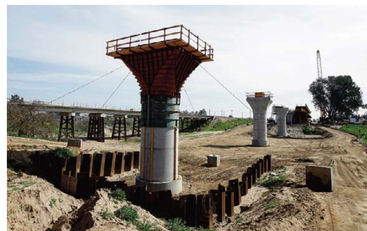
The supports for a 1,600-foot-viaduct to carry high-speed rail trains across the Fresno River are seen under construction near Madera, Calif. —AP
