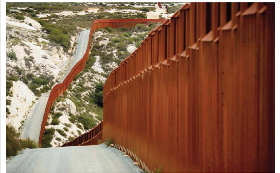
Photo shows a section of the border fence on the US/Mexico border in Tecate, California. — AFP
