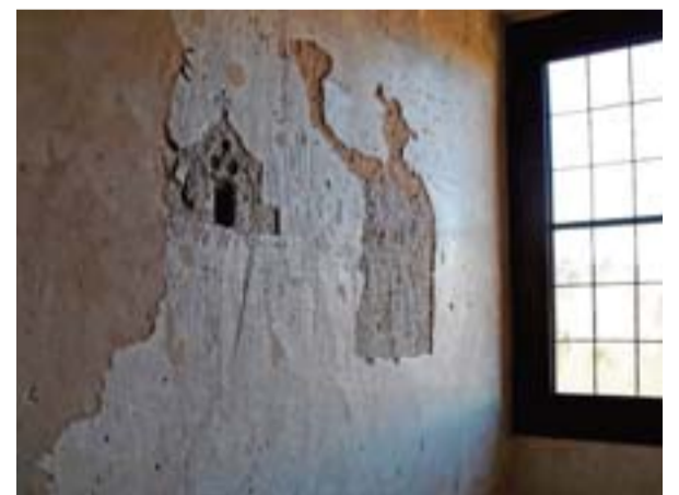
Photo shows graffiti and other markings left behind by prisoners locked in the Aljaferia tower in Zaragoza, Spain, during the Spanish Inquisition.
