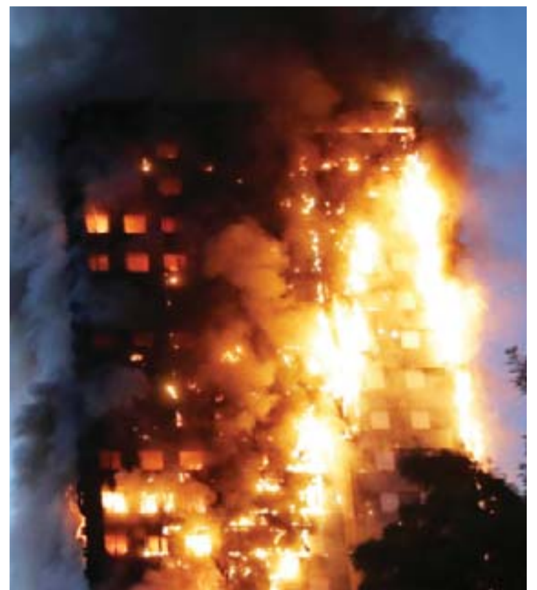
LONDON: Fire engulfs Grenfell Tower, a residential tower block yesterday in west London. The massive fire ripped through the 27-storey apartment block in the early hours of yesterday, trapping residents inside as 200 firefighters battled the blaze. — AFP
