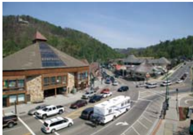
A fire-damaged building overlooks cars driving through downtown Gatlinburg, Tennessee.
