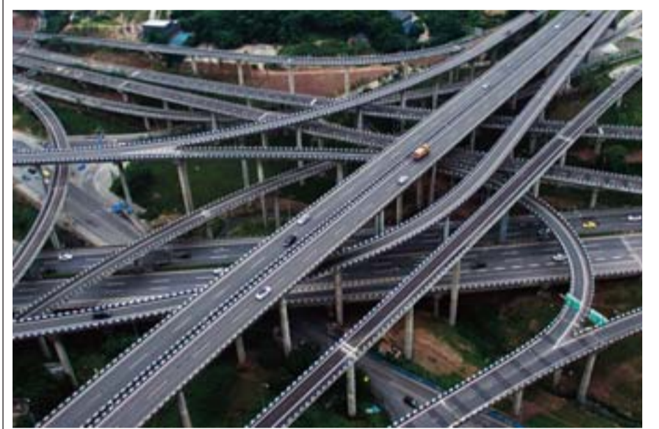
CHONGQING: This picture taken on June 3, 2017 shows motorists driving on an interchange in Chongqing, southwest China. The interchange is made up of five layers, 20 ramps and goes in eight different directions. —AFP
