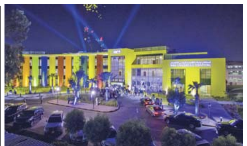
The National Bank of Kuwait Pediatric Hospital.
