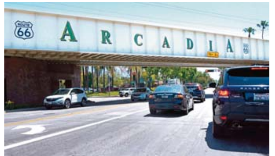
Route 66 signs on an overpass above Huntington Drive in Arcadia, California.
