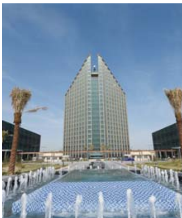
The new building of the Public Authority for Applied Education and Training (PAAET).
