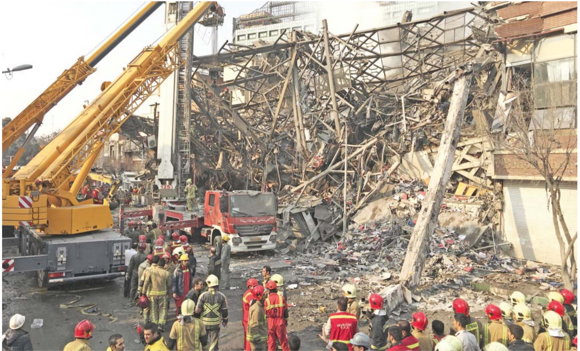
TEHRAN: Iranian firefighters work at the scene of the collapsed Plasco building after being engulfed by a fire, in central Tehran, Iran, yesterday. — AP
