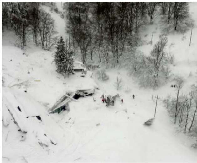
ITALY: An aerial view of the Rigopiano Hotel hit by an avalanche in Farindola, Italy, yesterday. — AP
